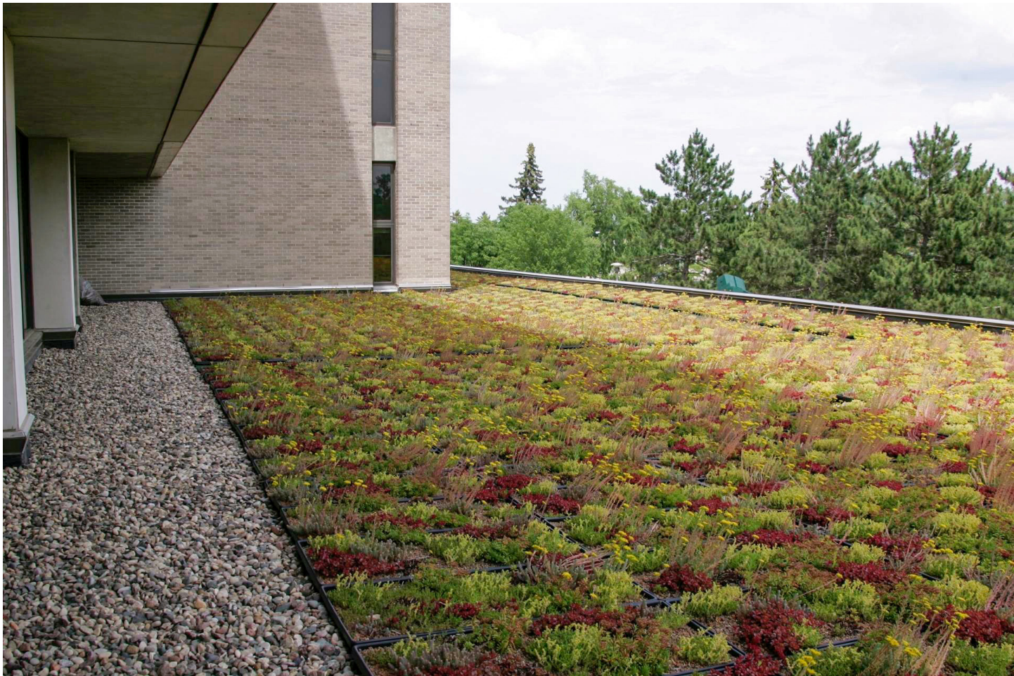
Existing Albertson Hall Green Roof
